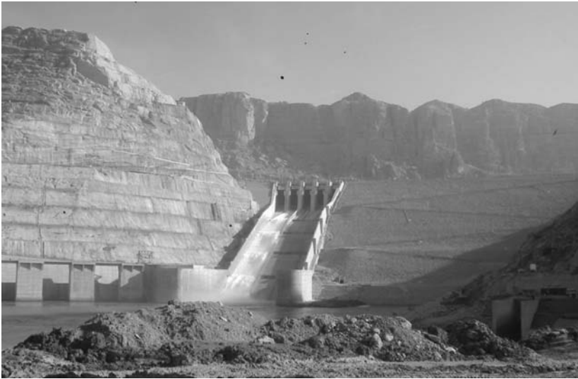
Figure 17.17 View of hydroelectric plant, the powerhouse cavern is inside the mountain on the left of the dam
